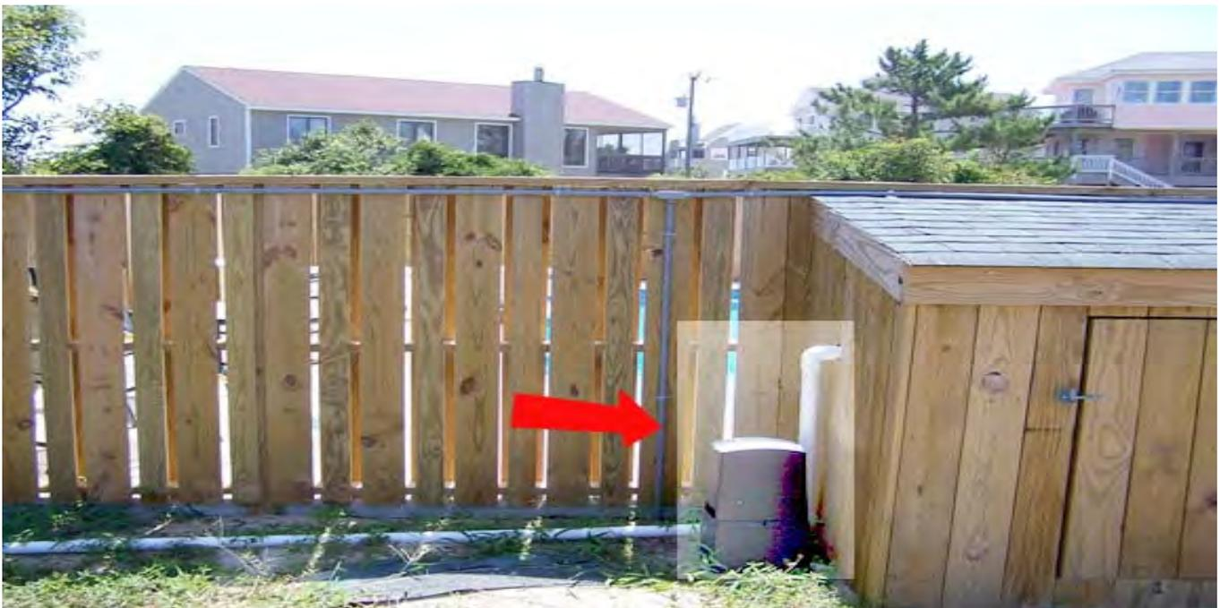
This barrier is 5 feet high and the lowest part of the pool equipment shed is 4 feet high. The horizontal members are spaced less than 45 inches apart so the verticals are spaced no more than 1 ¾ inches and the electrical conduit is OK. Problems: the optical lighting unit and the plumbing pipe location assist in climbing the barrier.
