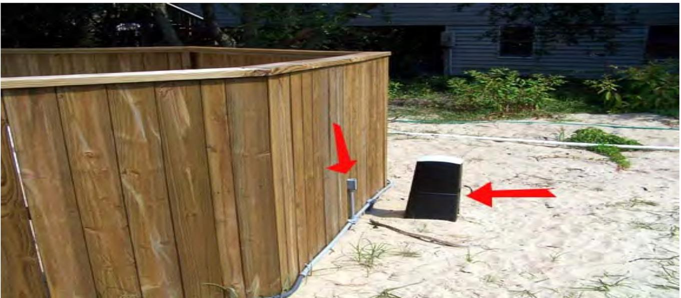
This barrier meets the minimum 4 feet height and barrier wall construction requirements but the location of the optical lighting equipment and the electrical device box provide assistance in climbing the barrier thus violating the provisions of **Section AG105.4 Prohibited Locations**.
