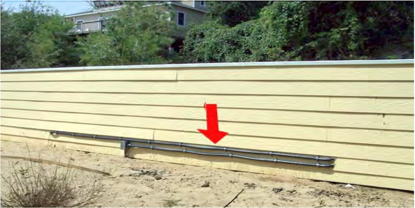
This barrier is 4 feet high and would meet barrier requirements if not for the electrical conduit. The conduit becomes a horizontal member and the location causes the horizontals to be less than 45 inches apart. This requires the conduit to be placed on the poolside, or on the top or bottom of the barrier to meet code.
