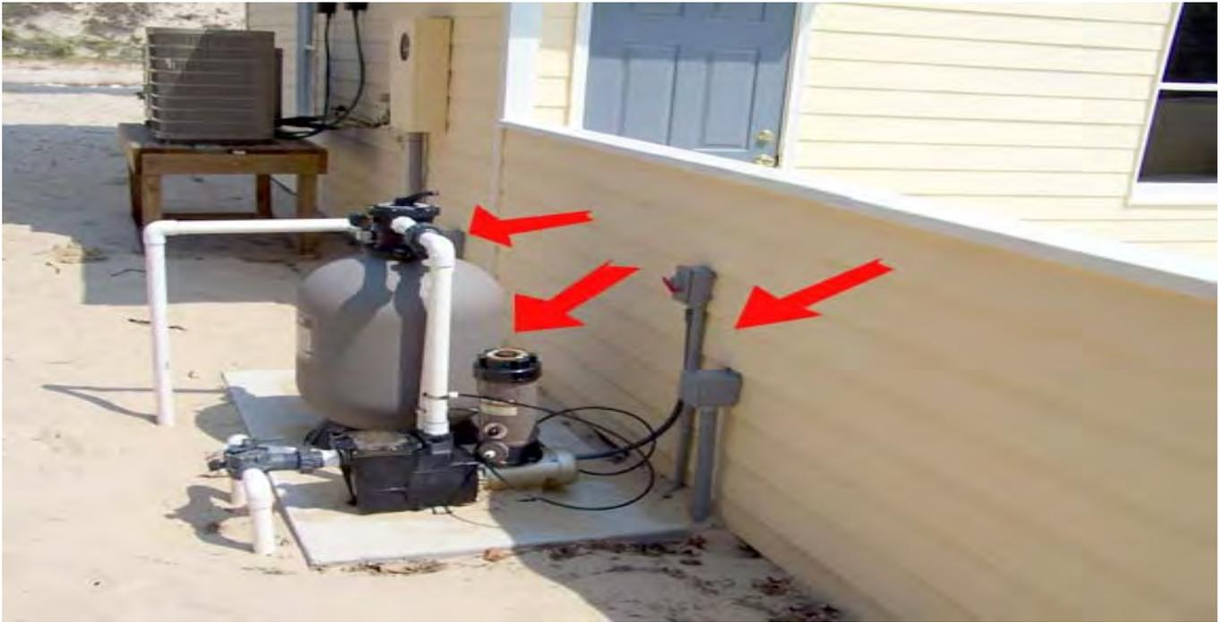
The above picture illustrates violations of **Section AG105.4 – Prohibited Locations**. The placement of this pool equipment and supporting electrical wiring help aid in climbing the barrier.
