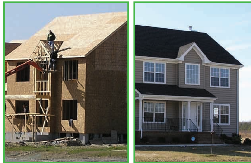
Shingle Landing - Before and After
